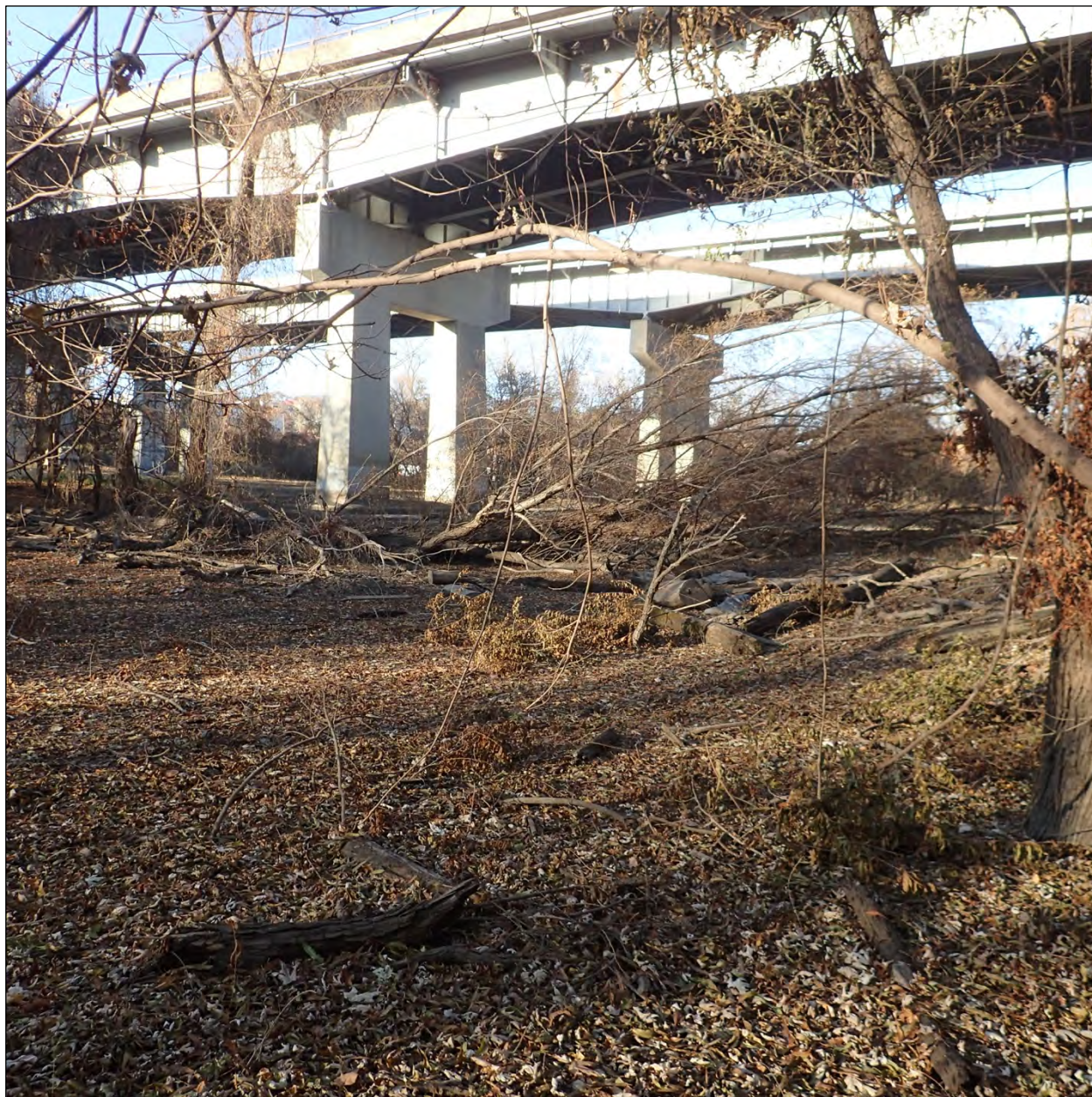
Figure 23. Continuous span I-70 girder bridge at the northeast end of the APE.
