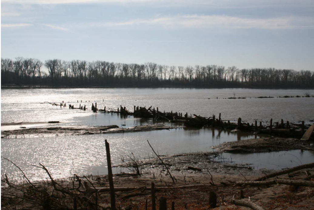
Figure 4 Pile dike on the Missouri
